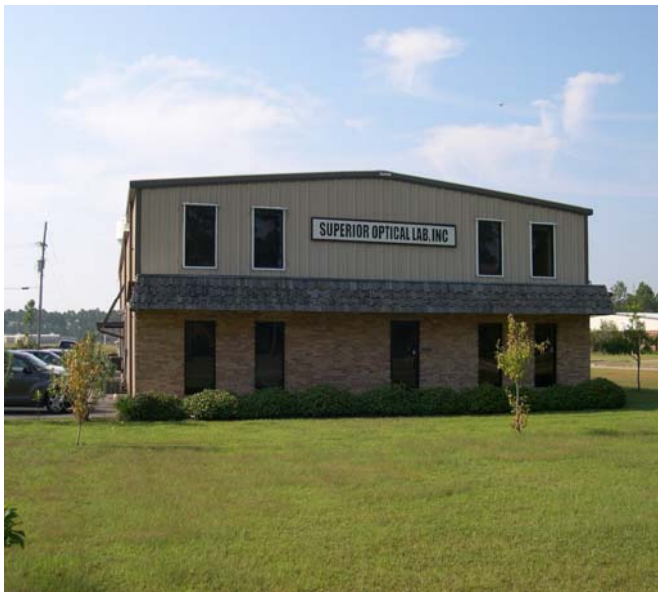
Superior is located in a light industrial park in Ocean Springs, Mississippi. Their building is situated on one acre of land and is 7000 sq. ft. Currently they have a 4000 square feet of existing lab, 2000 square feet for administration and 1000 square feet for future expansion
